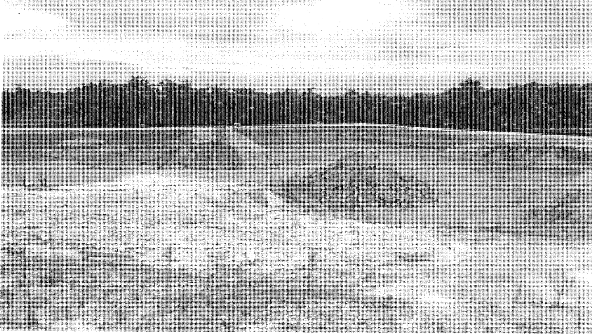
Close up of Pond 1 rim, showing high water mark indicating near-overtopping from prior storm. (July 23, 2021)
