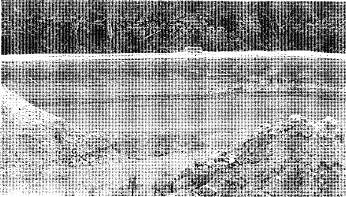
Close up of Pond 1 rim, showing high water mark indicating near-overtopping from prior storm. (July 23, 2021)
