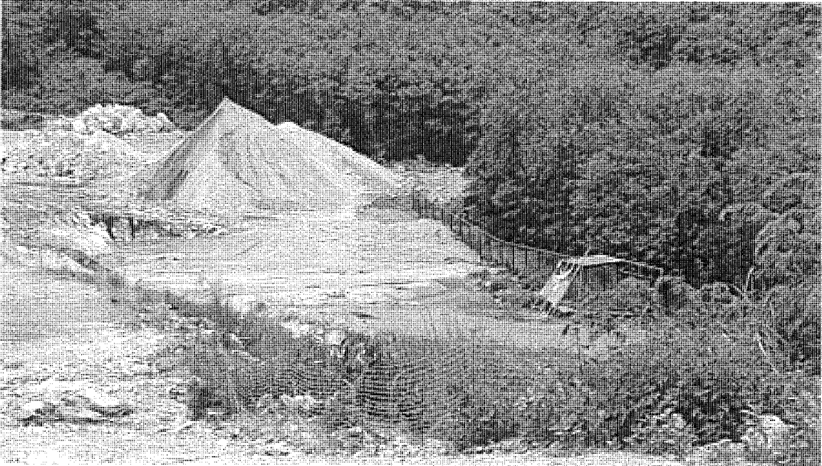
Close-up of area that appears to be a large, unprotected off-site discharge toward Marbo Cave area. Note large delta-type formation of sediments, indicating long-term history of discharge. (July 23, 2021)
